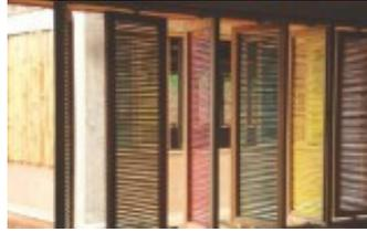
*An innovative facade made using pivoting bamboo shutters to allow the most natural light and ventilation. Photos: Arup International Development and Sabre Trust.*
